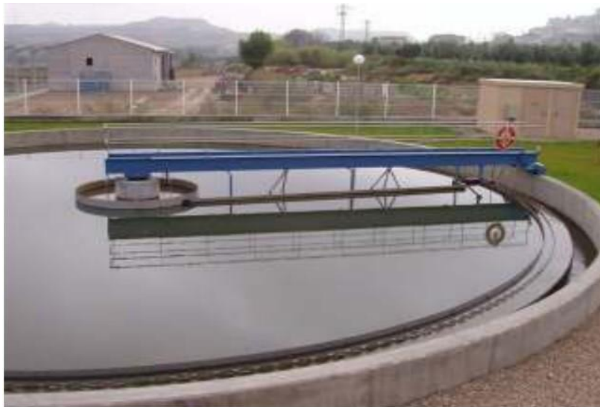
Figure 36: Primary clarifier
