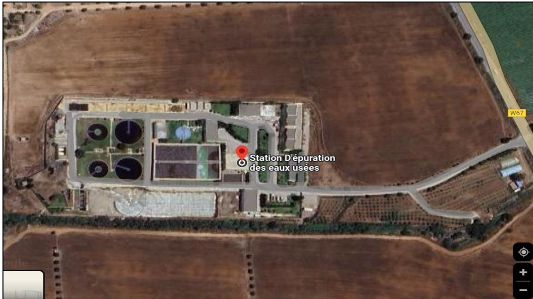
Figure 31: location of the station with google maps
