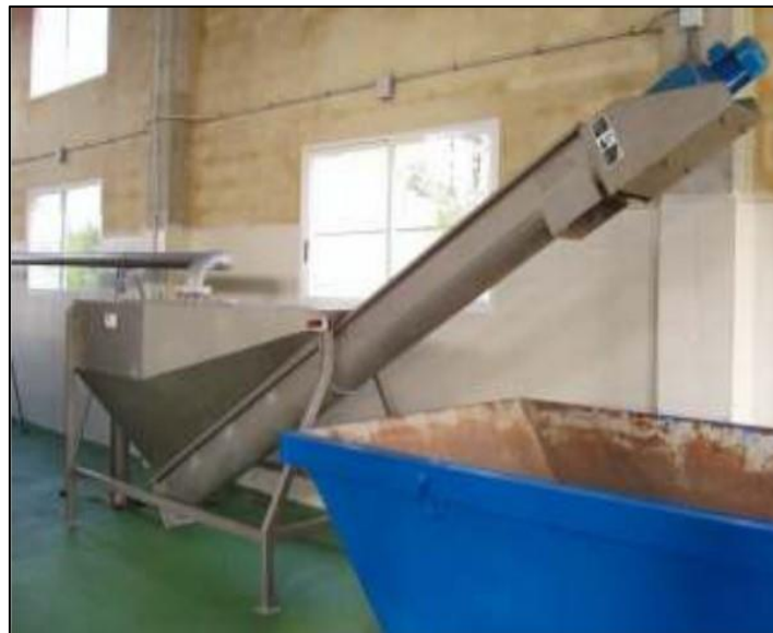
Figure 33: Sand Classifier
