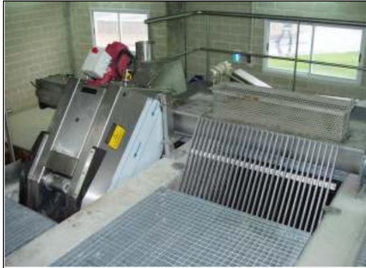
Figure 32: Rough and manual grid
