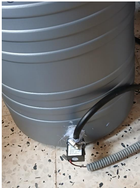
Figure 26 water source tank & inlet pump
